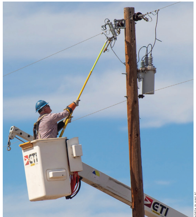
Elbie Wilson, who has 22 years of experience at North Plains EC, takes a single-phase recloser out of the loop and places the downstream line behind the fuse as part of the co-op’s preparations for a major wind event in March.
